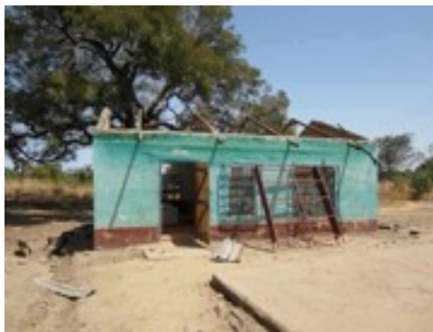
Roof removed ready for raising the sides
