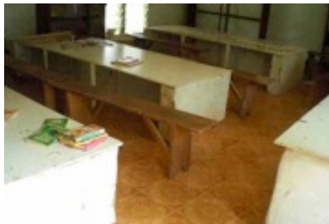
The flooring completed
