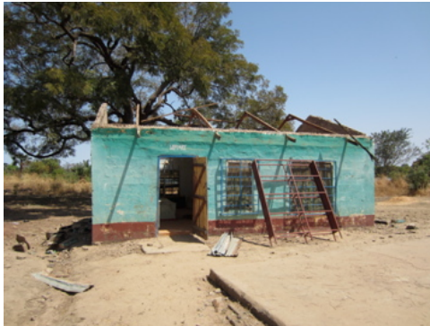
Roof removed ready for raising the sides
