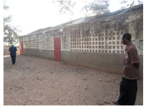
Classrooms to be re-roofed at Sololo basic cycle school
